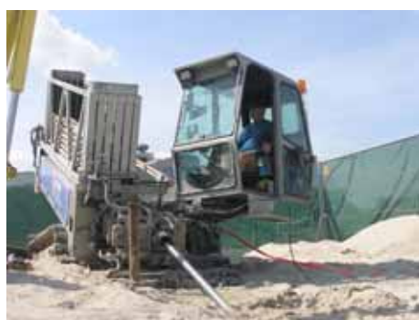
The GRUNDODRILL 15 N during pipe installation.
