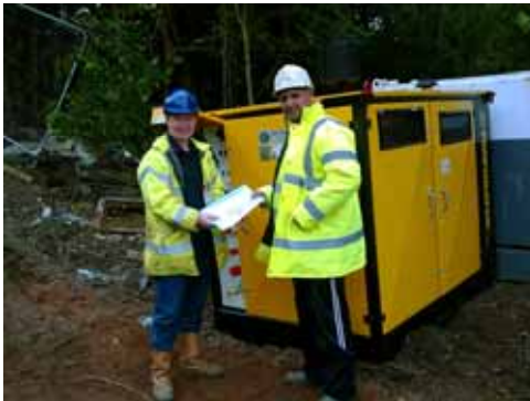
Taking delivery of the HS80 Power Pack.
