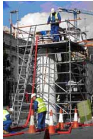
A typical Insituform CIPP inversion tower.
