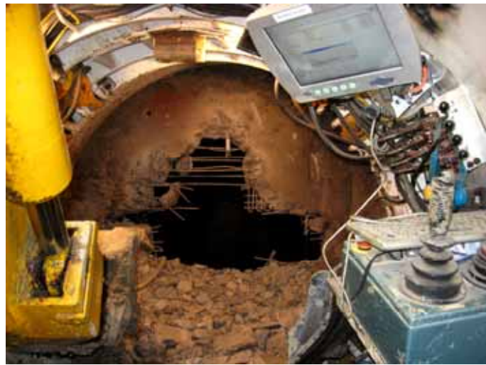
The Herrenknecht MH3 Open faced backacter unit completes holing on the first of the Sidcup drives.
