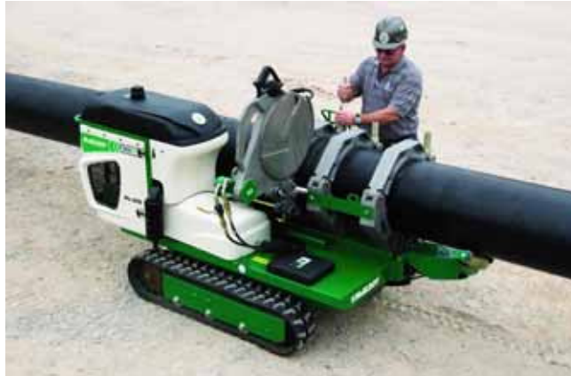
A McElroy TracStar618 pipe fusion system operating in the field.
