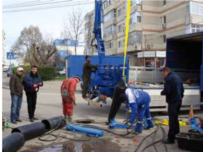
The Expandit system working on a project in Romania.
