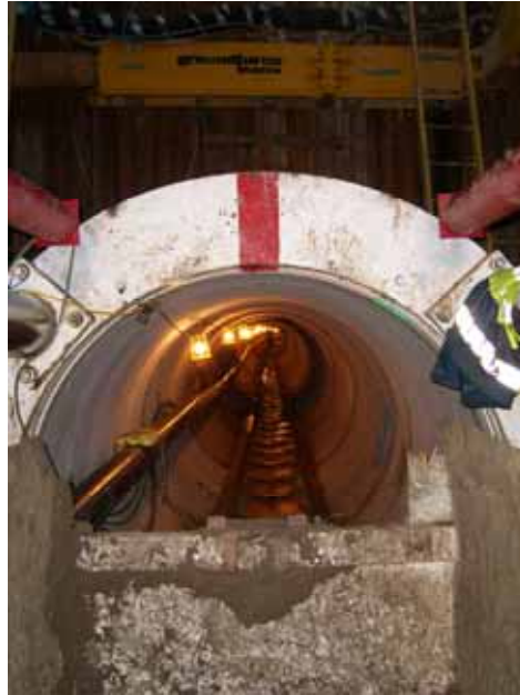
A view along one of the curved Sidcup pipe jacked storage tank drives from the launch cofferdam looking through the shove ring and over the muck skip.
