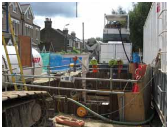
The surface setup at the start shaft for the Sidcup curved drives.
